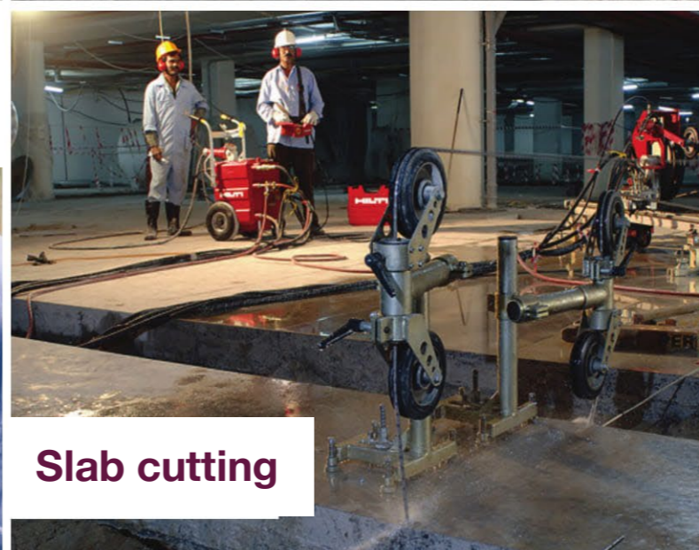
Making large opening in concrete
