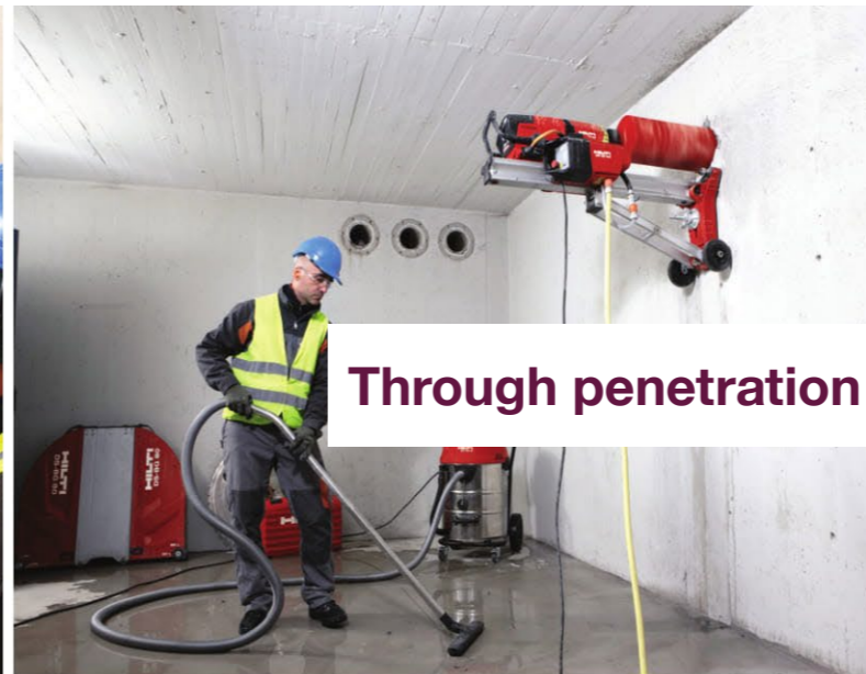
Angular core cutting for drainage pipes
