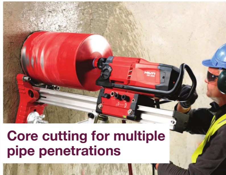
Small wall opening
